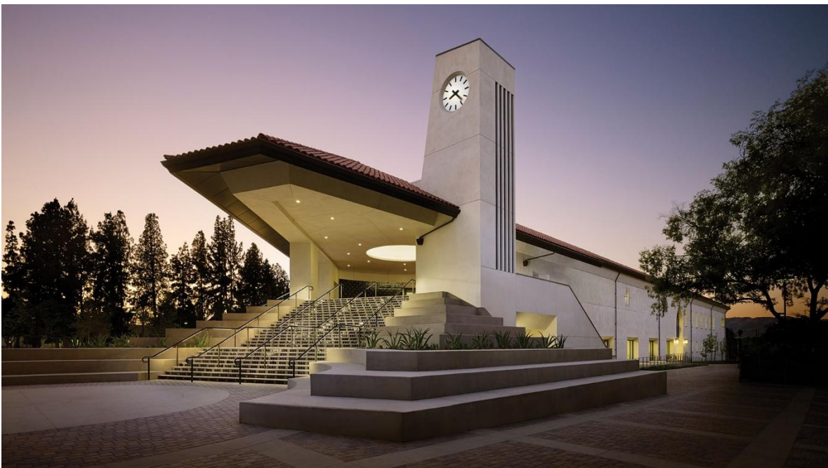
Figura 26. Fachada principal de Pierce College Library/Learning Crossroads
